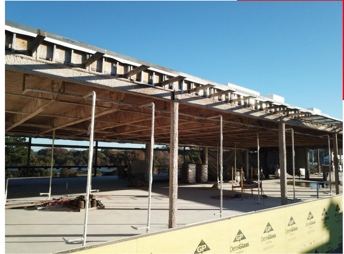
Fireproofing Progress at 4 th Floor of New Addition
