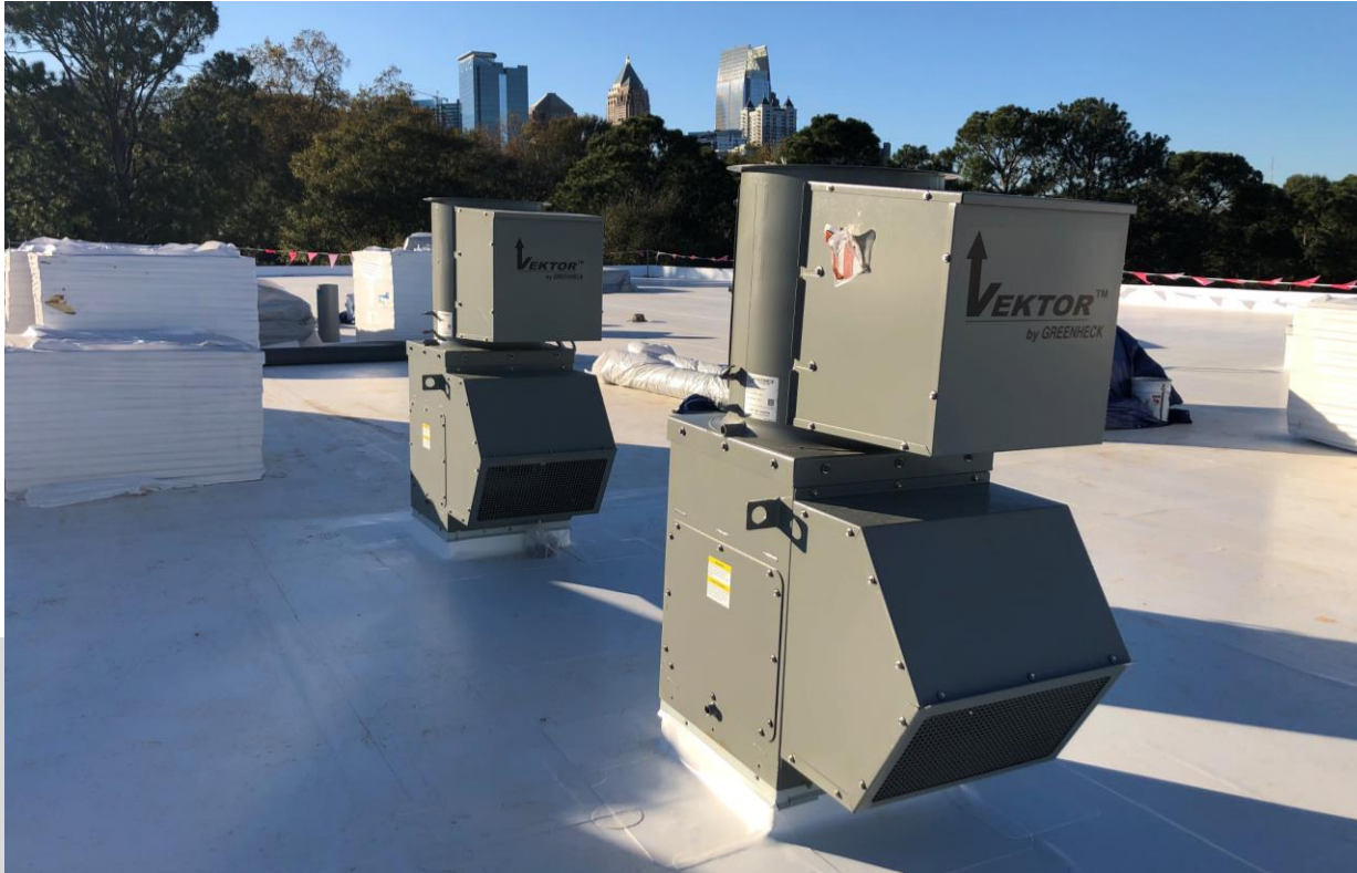
New Exhaust Fans Installed at New Addition Roof
