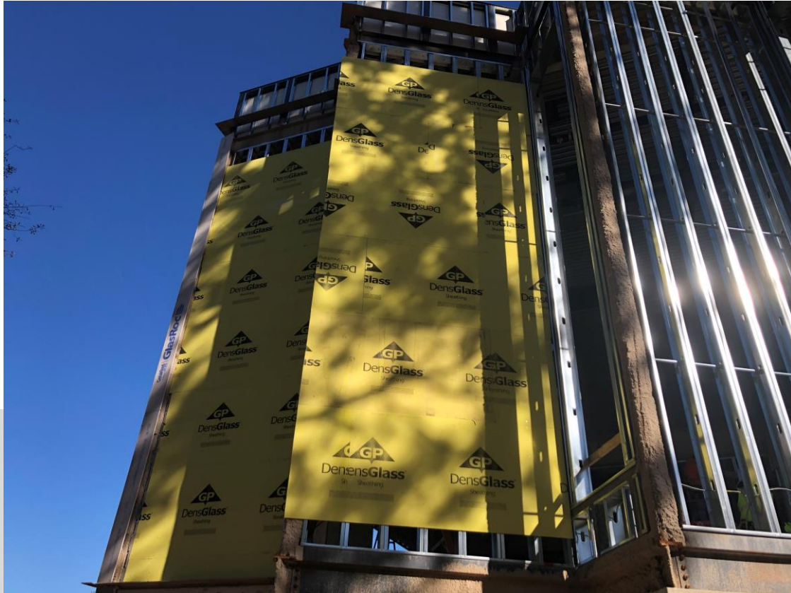
Exterior Sheathing installed at New Addition Media Center Wall
