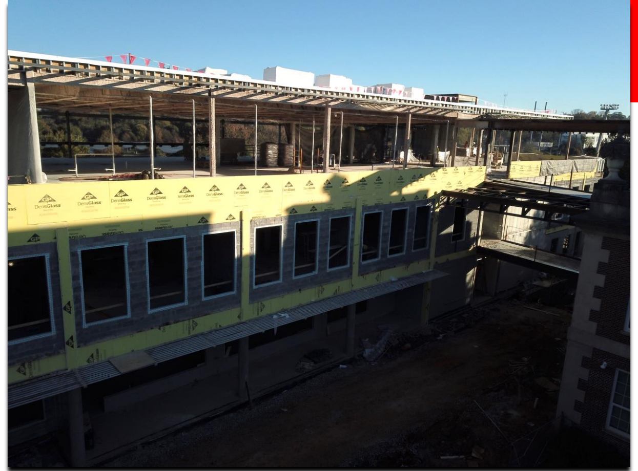
Exterior Sheathing Completed at South Side of New Addition
