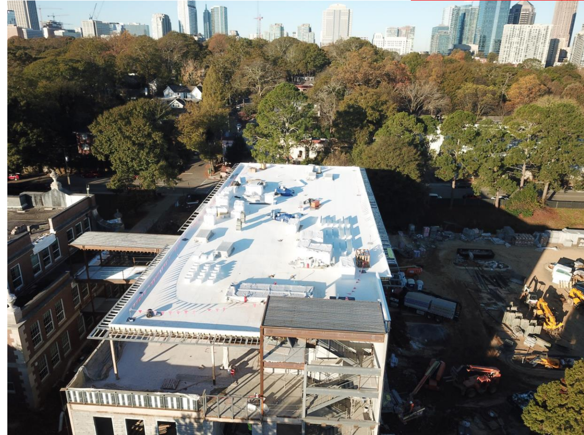
New TPO Roof Installed at New Addition and Rooftop Curbs Set for new HVAC Units
